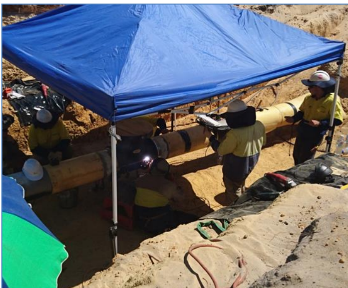
Live Line welding of Stopple Tee
