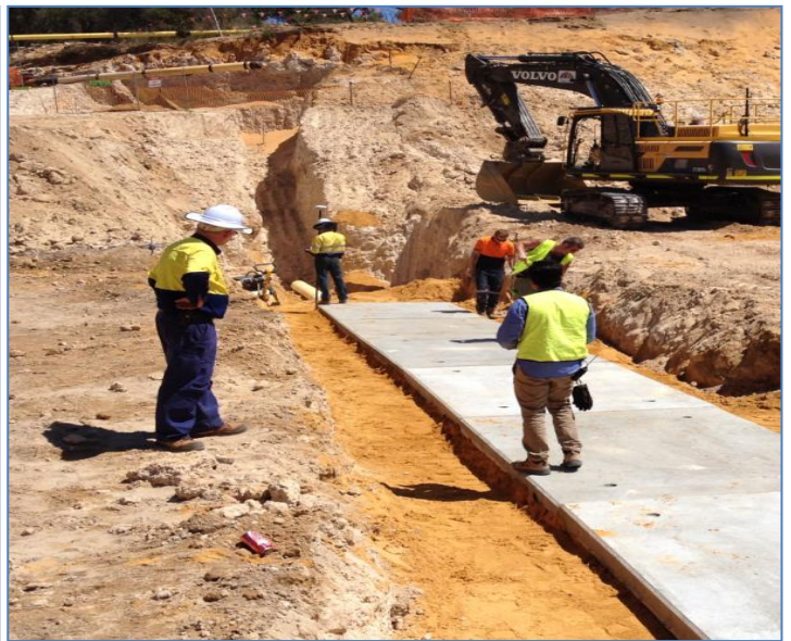
Survey and Installation of Pre-cast Concrete Panels
