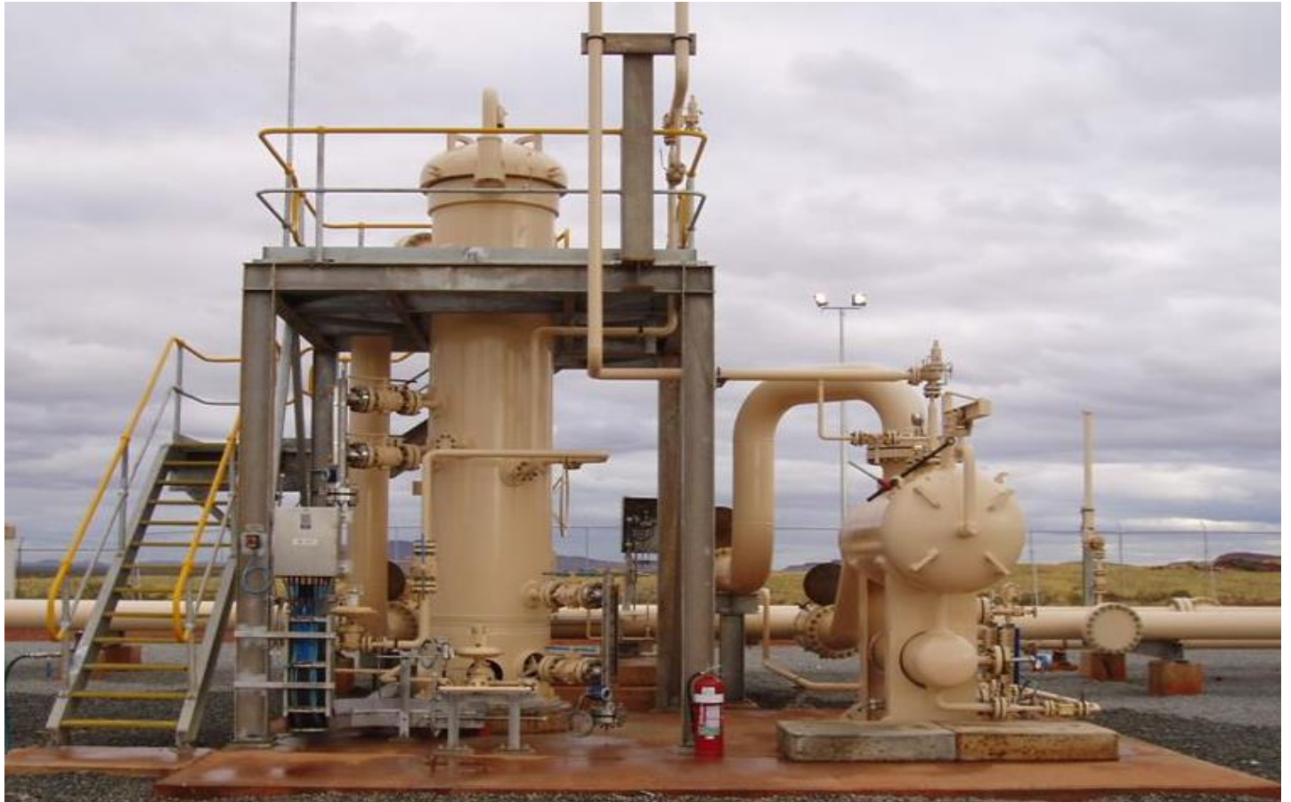
APA Group – Wyloo Compressor Station Inlet Coalescing Filter Vessel installed on site
