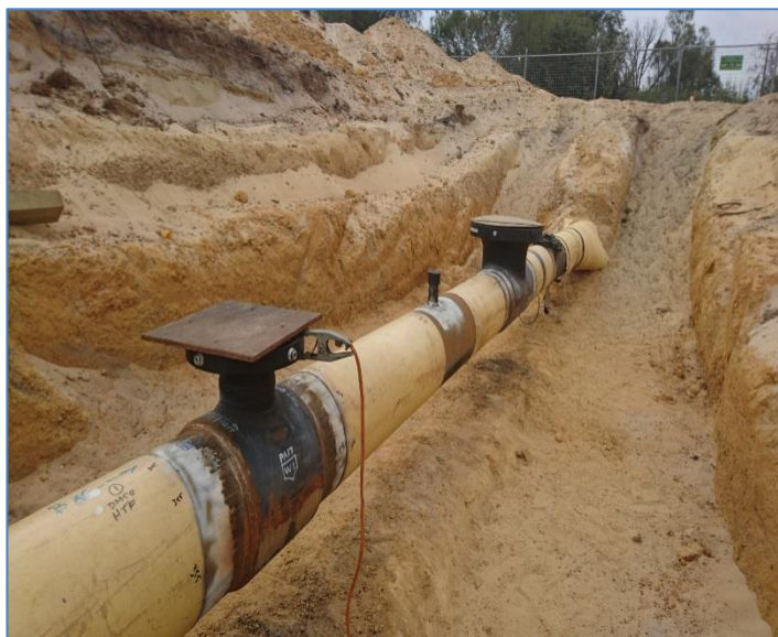
Completed Hot Tap Tees Northern Excavation
